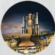
Encorp Strand Mall Kuala Lumpur, Malaysia.
